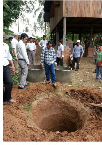
East Meets West staff inspect latrine construction prior to rings being installed. Photo credit: Paul Crawford
